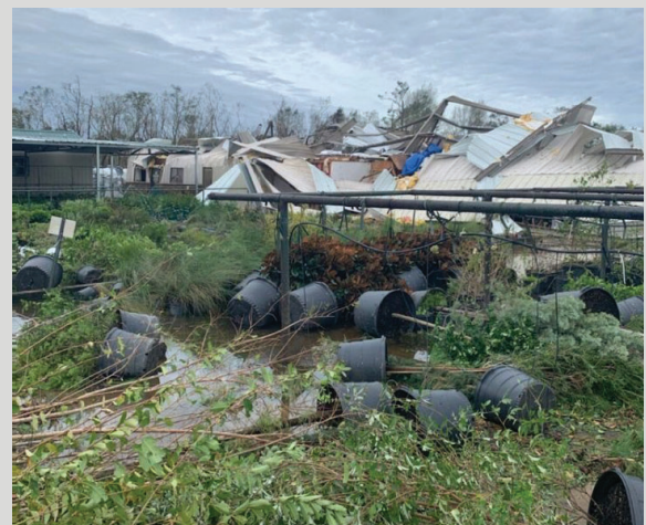
Heartbreaking destruction at Landscape Management Service in Lake Charles
