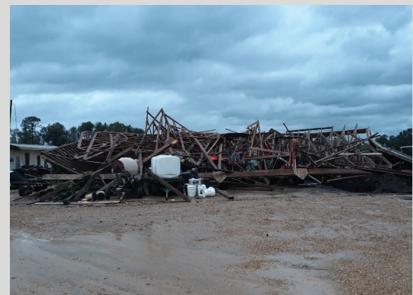
Damage at Thaico Nursery in Forest Hill
